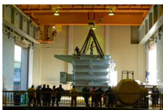
Replacement of Generators for Transformers at Steenbras Power Station: Electrical Engineering Services
